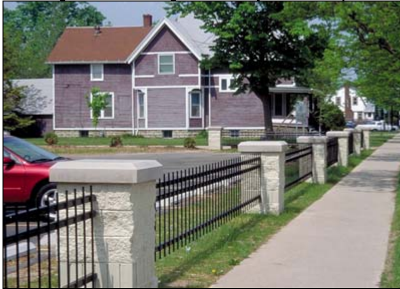
Figure 12-6: Fencing and Masonry Walls Example
