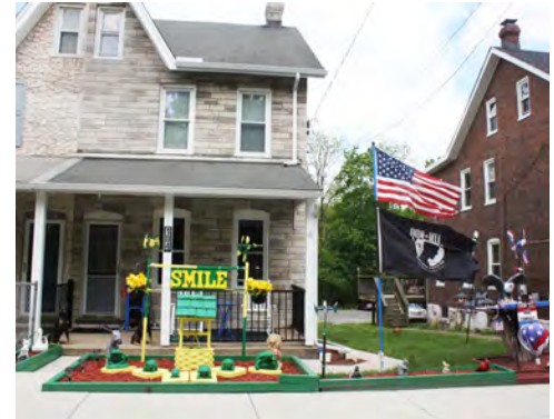
The MDR designation generally features single-family detached dwellings and twins on smaller lots than those designated LDR. This example is located along North Brandywine Avenue.
