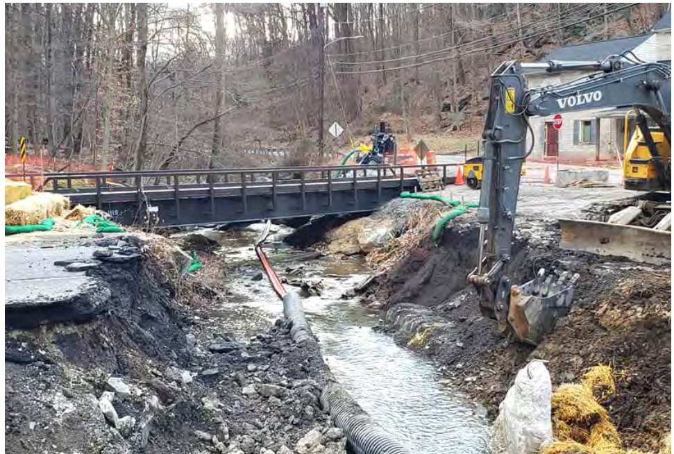
From 2019 to 2020 the deteriorating South Brandywine Avenue bridge spanning Dennis Run was replaced utilizing funding in part from the Chester County Department of Community Development. Image courtesy of the Borough of Modena.
